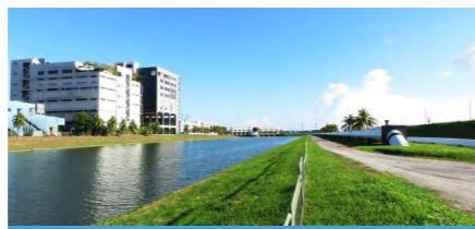
River Water Level Monitoring
