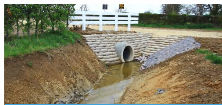
Irrigation Canal Water Measurement and Monitoring
