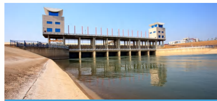
Pump Station Monitoring
